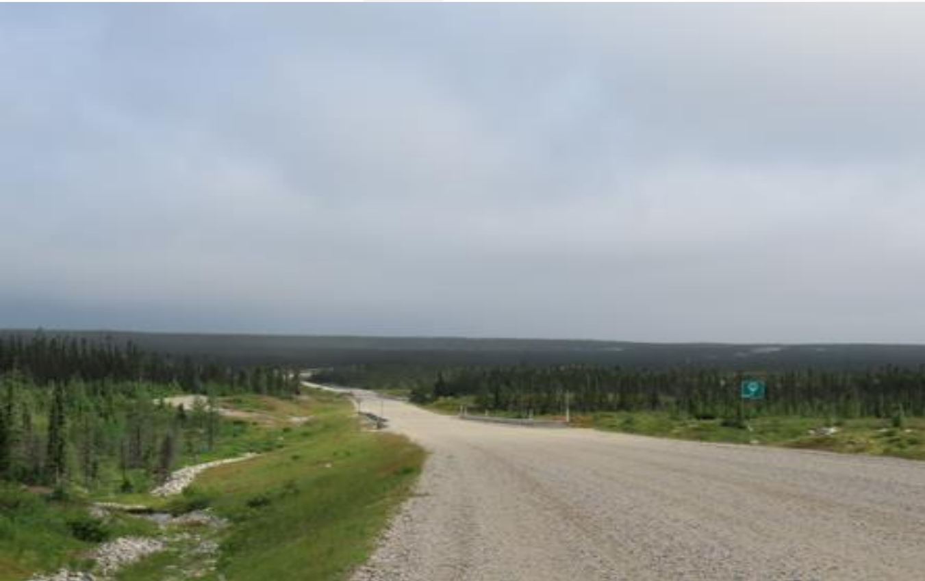
Route 167 – An All Weather Road
