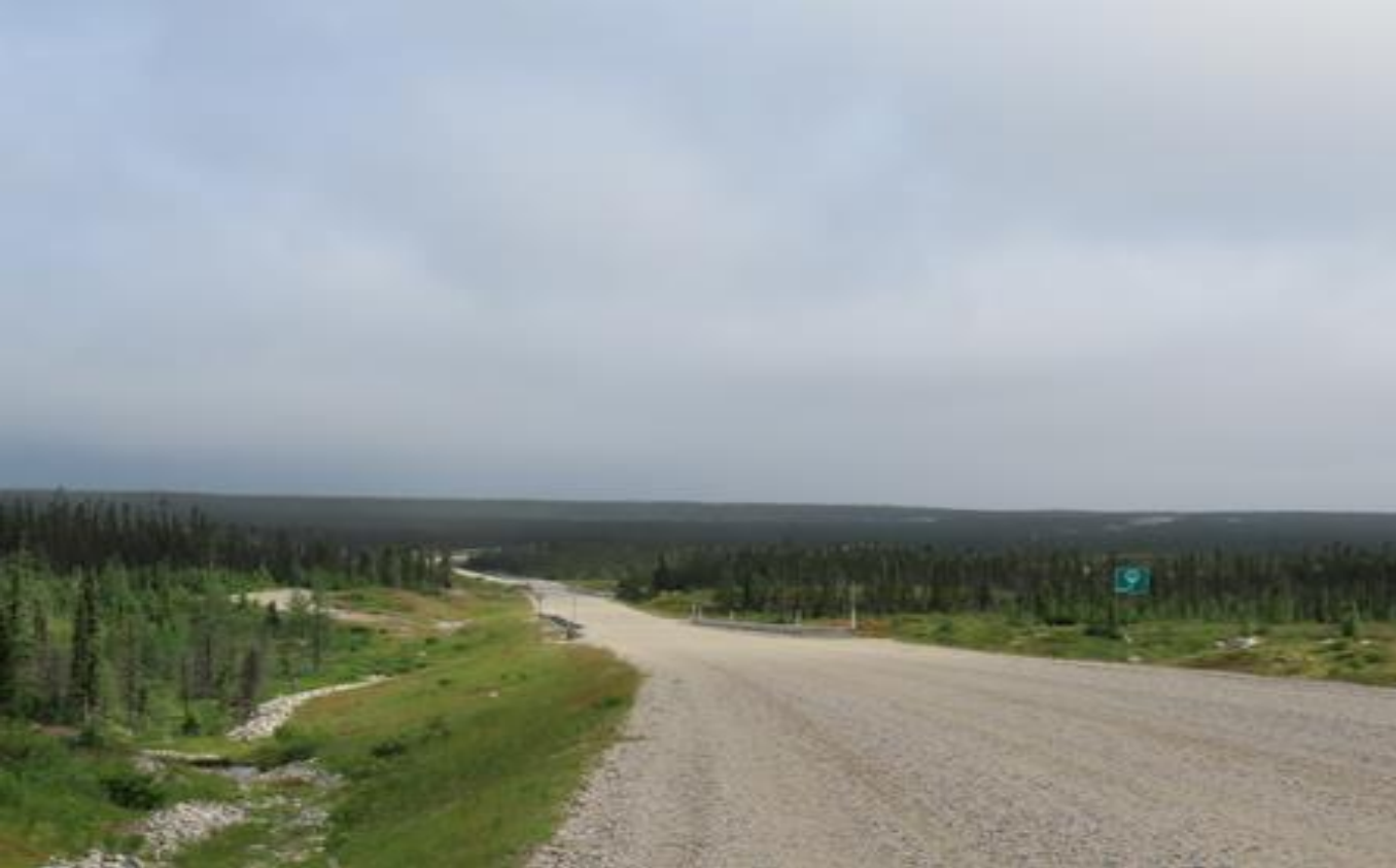
Route 167 – An All Weather Road
